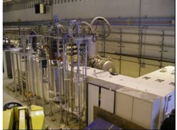
Figure JRA1.10.6: Re-installation of the helium compressor and vacuum pumping system (left) and the CryHoLab area (right).
